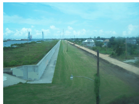
The levee, now repaired, breached by Katrina
